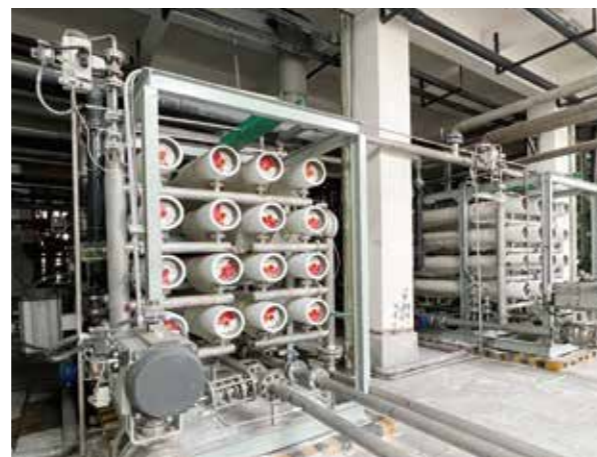
A 20000t/d zero discharge project for iron phosphate production wastewater from a certain enterprise in Henan Province (Phase I + Phase II)
